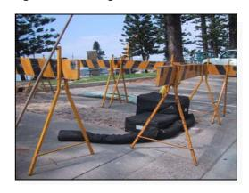
FilterBales & socks preventing sediment run-off from construction site
